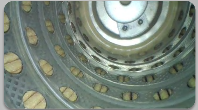
Lubrication Filter Inspection Using a 3.9mm VQ2 039 1500 4
