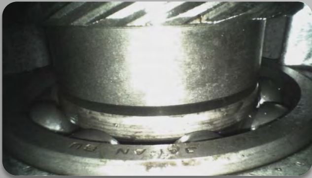
Gearbox Inspection Using a 6mm VQ2 060 1500 4
